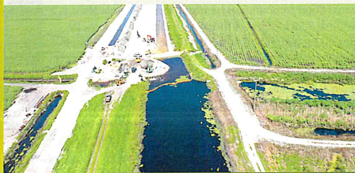
G-341 Conveyance & Related Improvements; Segment #4 Construction. (Photo by SFWMD)
